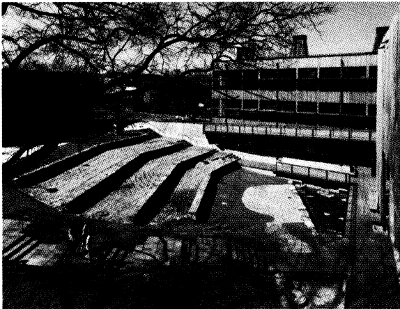
The plants in the terraces of Sidwell's subsurface-flow constructed wetland (left) are expected to grow in over the summer. Subsurface wetlands (above) control odors and environmental hazards by keeping water underground.
